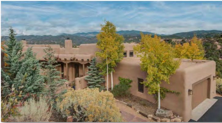
84 CIRCLE DRIVE COMPOUND
